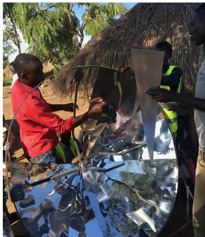
Assembly of the solar cooker SK14
