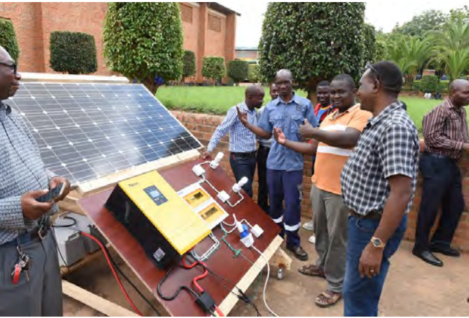
Commissioning of the photovoltaic hybrid system by the participants
